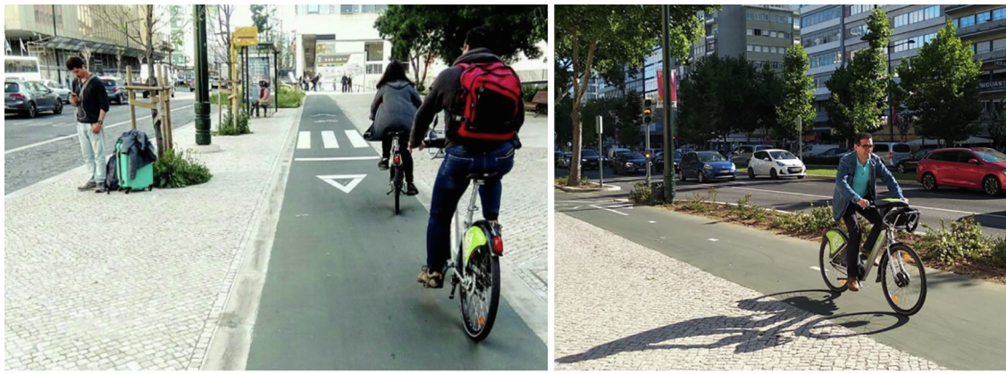
Fig. 6. Segregated bicycle infrastructure at the sidewalk level, uni and bi-directional, respectively, in central Lisbon (photo credits: Sexta de Bicicleta – MUBi ).
